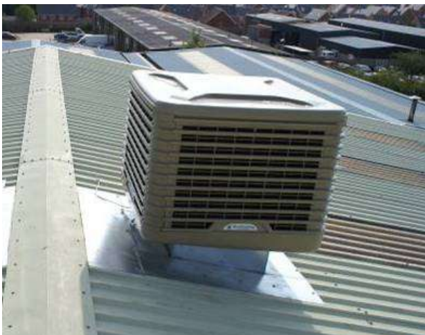
Figures 14 and 15. Photos of a typical rooftop ECPD installation. The weight of the cooler is supported on the underside of the roof.
