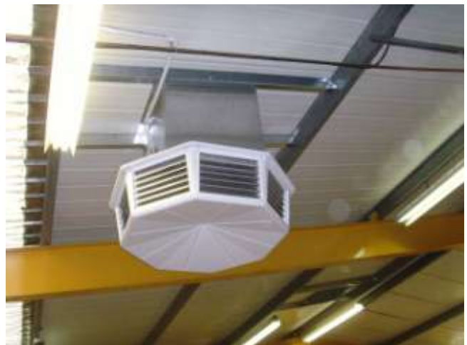
Figures 14 and 15. Photos of a typical rooftop ECPD installation. The weight of the cooler is supported on the underside of the roof.
