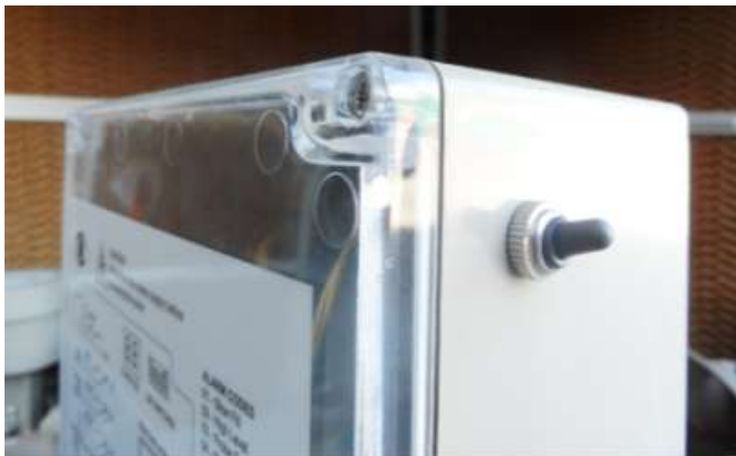
Figure 38. The test switch located on the side of the EcoCooler's main control box.
