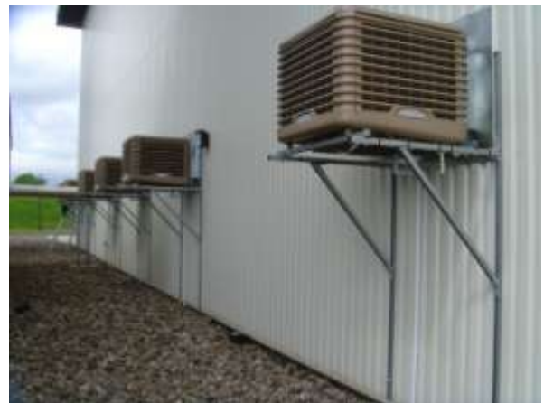
Figures 21 and 22. An image featuring dimensions and a typical ECPS mounted on a scaffold frame.
