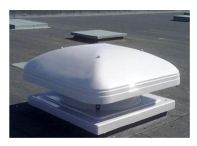
The Low Profile Cowls can be supplied with non-return shutters and bodyguards as standard.
